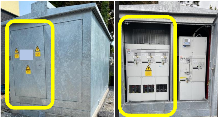
Figure 17: Example of Customer owned modular enclosure for MV Customer. DSO enclosure in yellow box.
