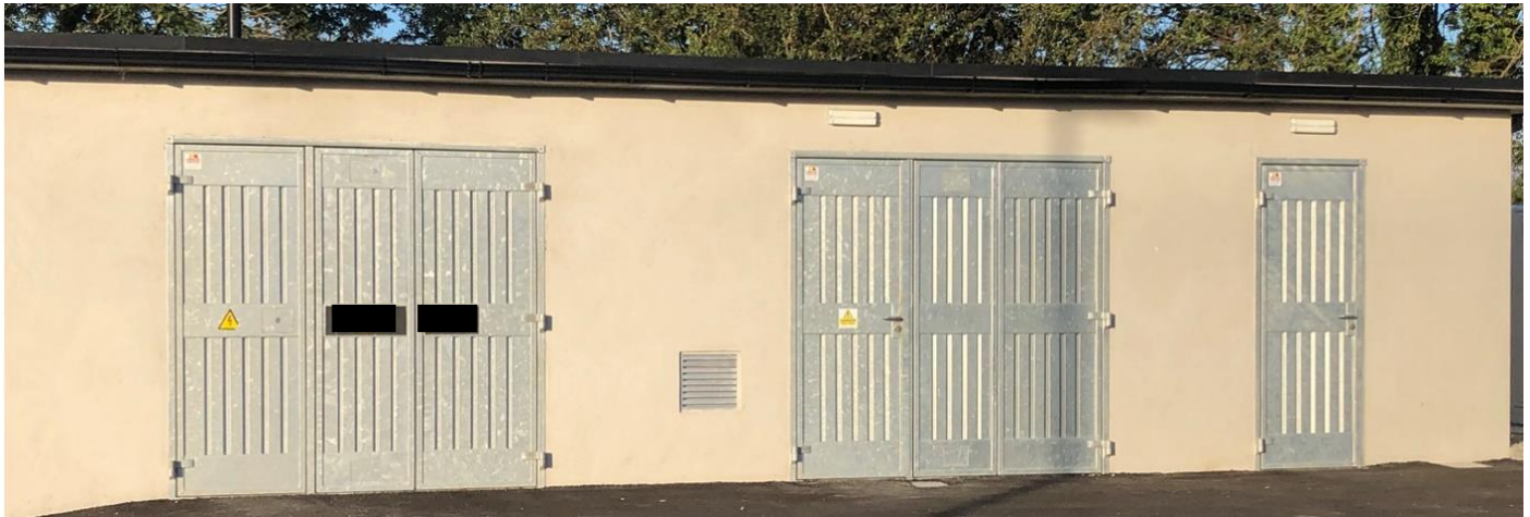
Figure 17: Example of Customer owned modular enclosure for MV Customer. DSO enclosure in yellow box.
